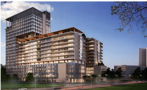
OUTRAM COMMUNITY HOSPITAL 10 Hospital Boulevard, Singapore
