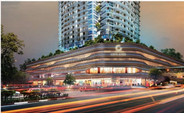
CITY GATE 371 Beach Road, Singapore
