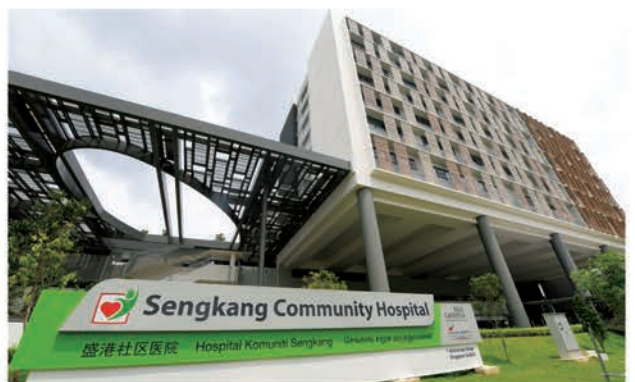
SENGKANG COMMUNITY HOSPITAL 1 Anchorvale Street, Singapore
